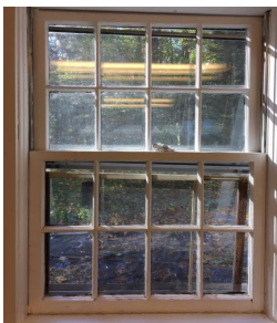
Check old windows for chipped paint.
